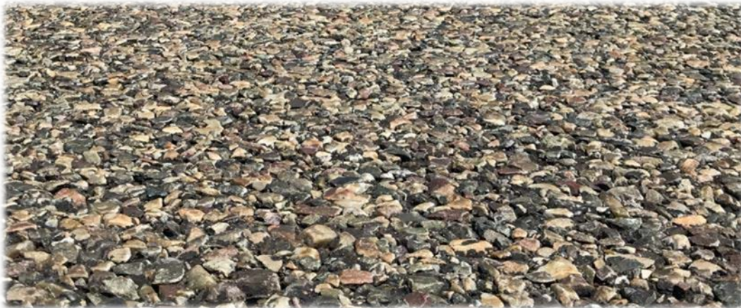
Figure 7. Close-up of typical exposed aggregate (1/2-inch) surface observed on the runway.
