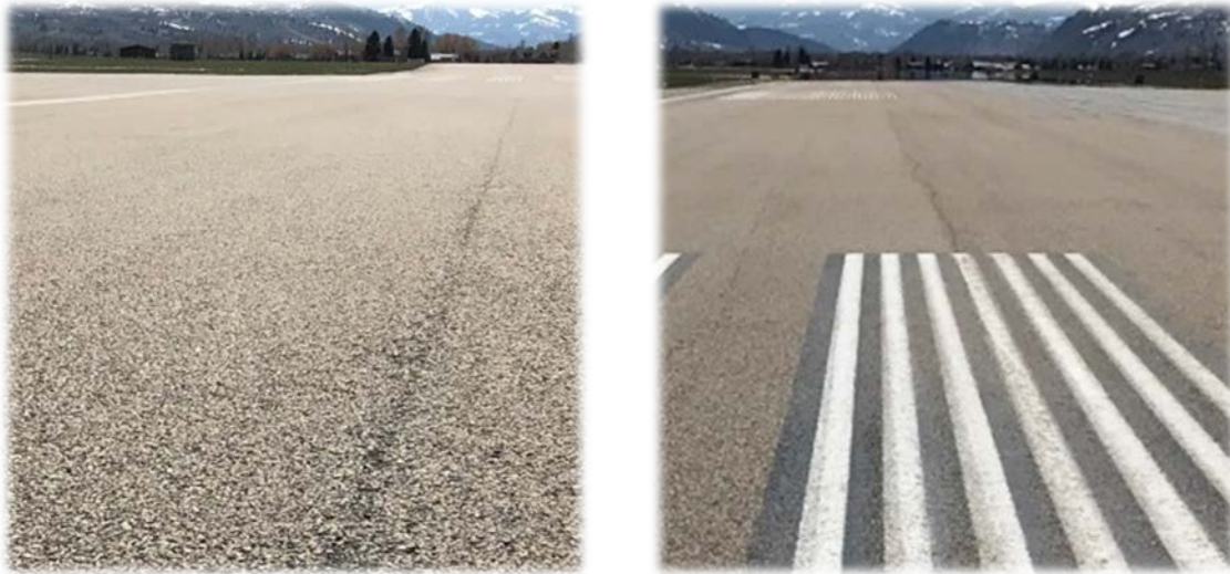
Figure 9. Example of deterioration at longitudinal paving joints.
