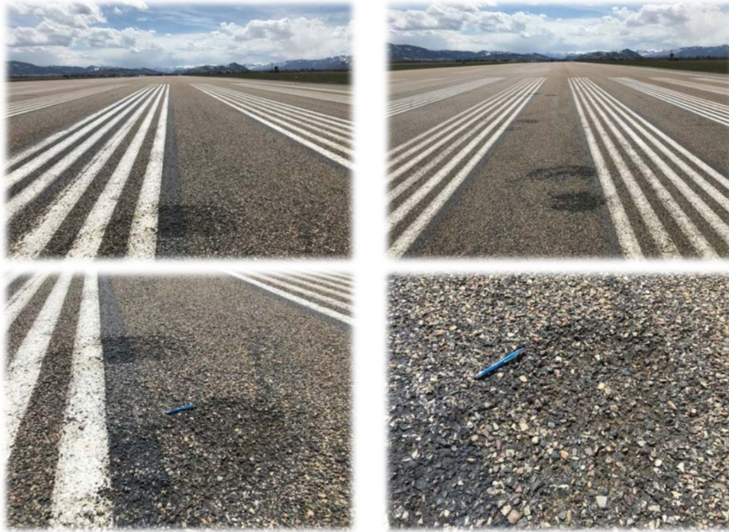
Figure 5. FR-PFC material loss from locked-wheel aircraft turning maneuvers.
