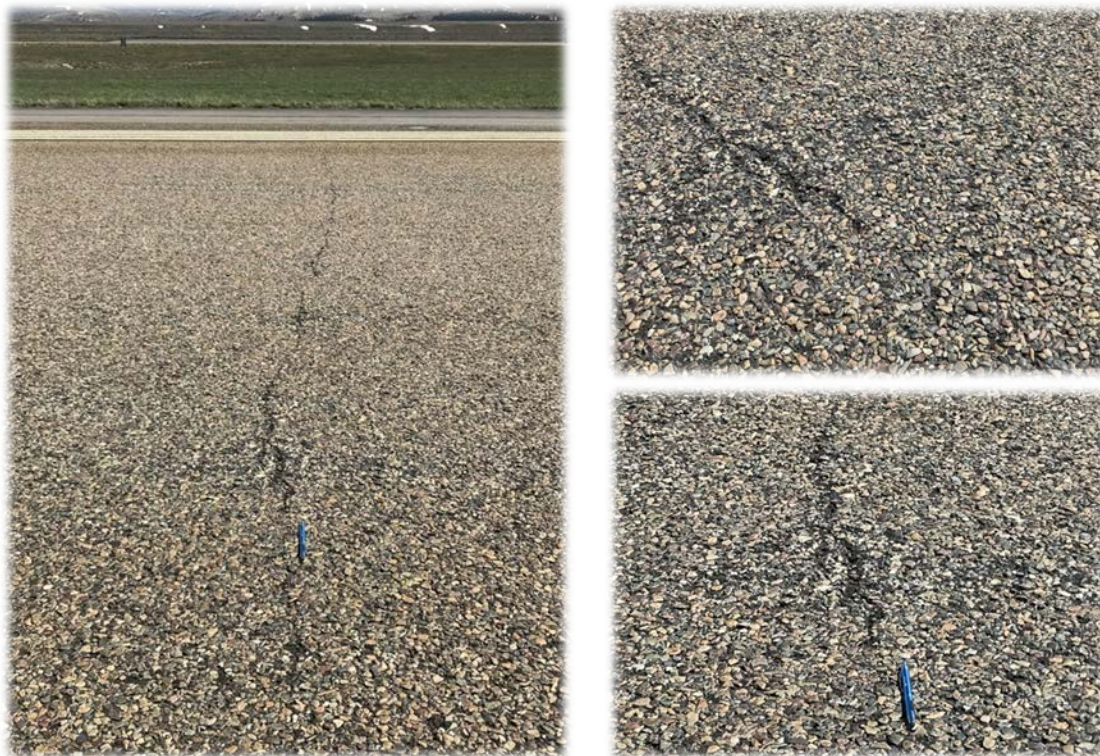
Figure 4. Low severity transverse cracking.
