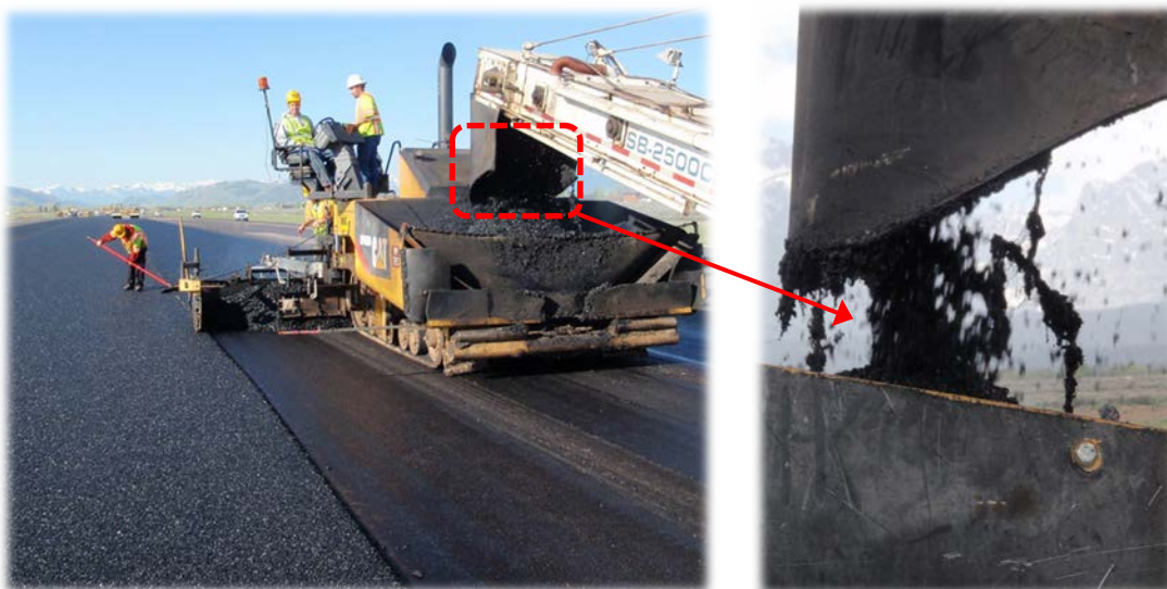
Figure 3. FR-PFC paving (left image) and close-up of blended aramid fibers (right image).
