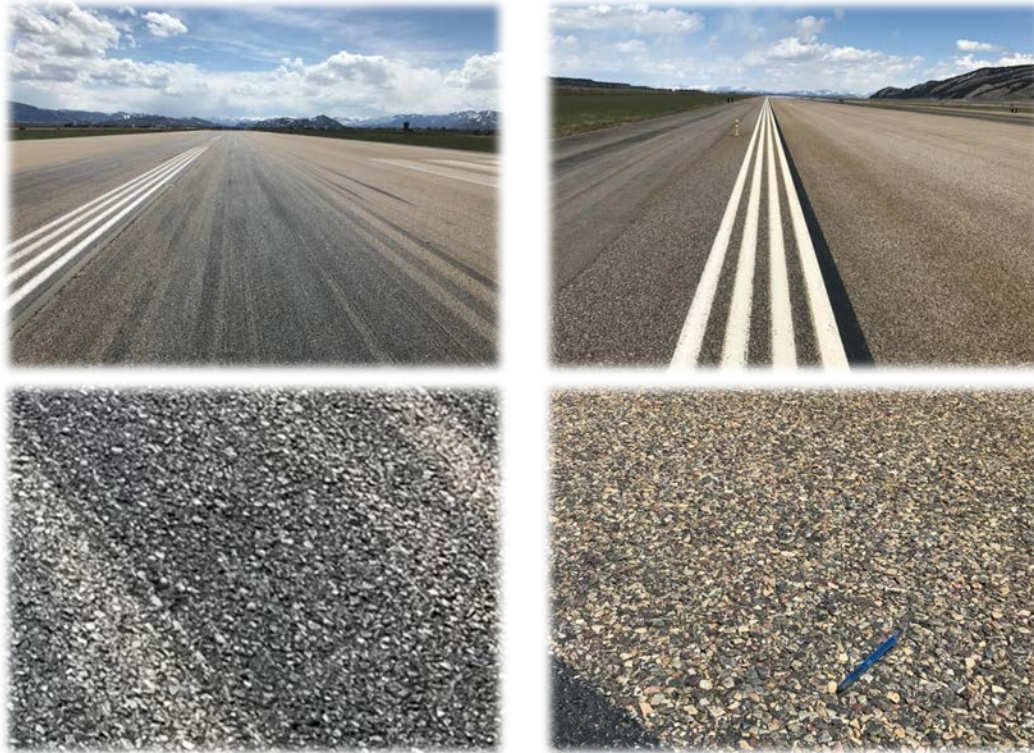
Figure 6. Example of centerline surface with rubber build-up (top-left image) edge surface (top-right image) and associated close-up of surfaces (bottom images).
