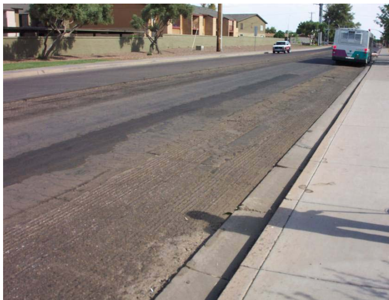
Figure 6 Surface Preparation by Milling off the Edge of the Pavement
