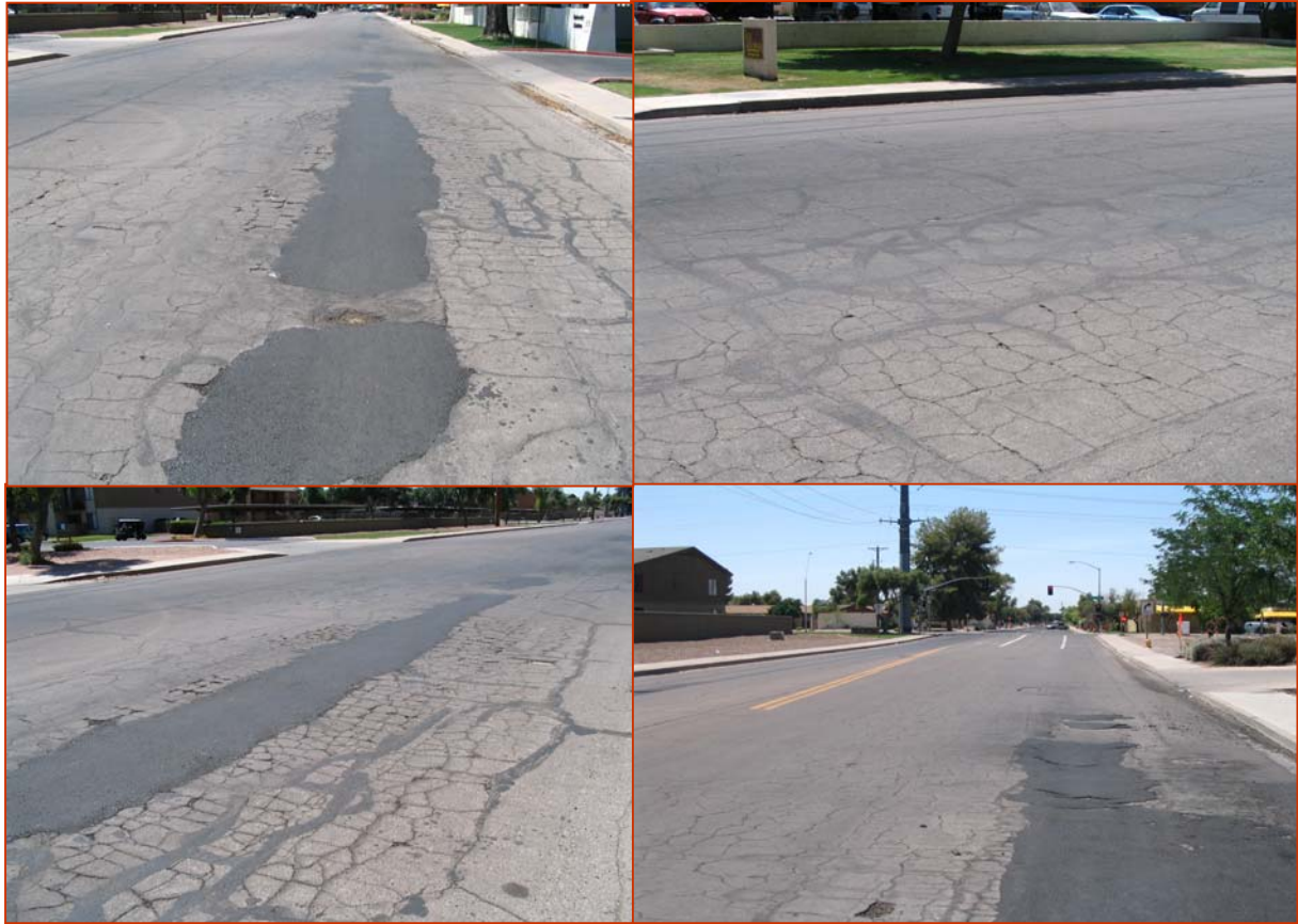
Figure 5 Pavement Section before the Fiber-Reinforced Asphalt Concrete Mixture Overlay
